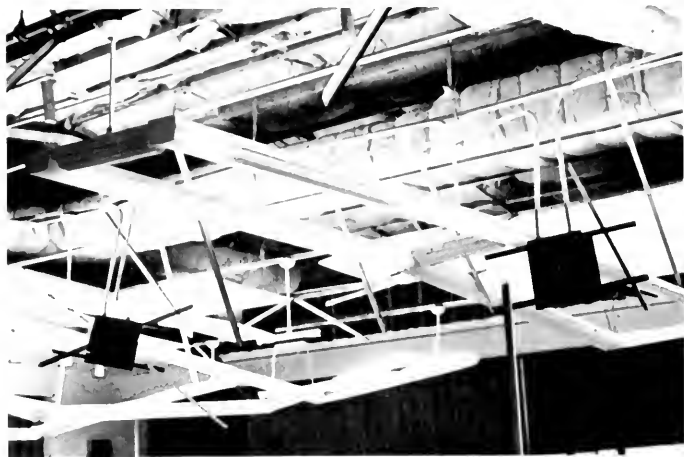
Photo 21. Soledad Canyon Elementary School. Damage to ceiling and light fixture in the multipurpose room.
